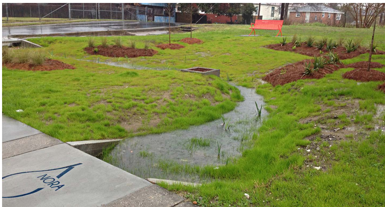
A storwater lot in Hollygrove collects runoff and allows it to enter the soil, courtesy Dana Brown & Associates.
